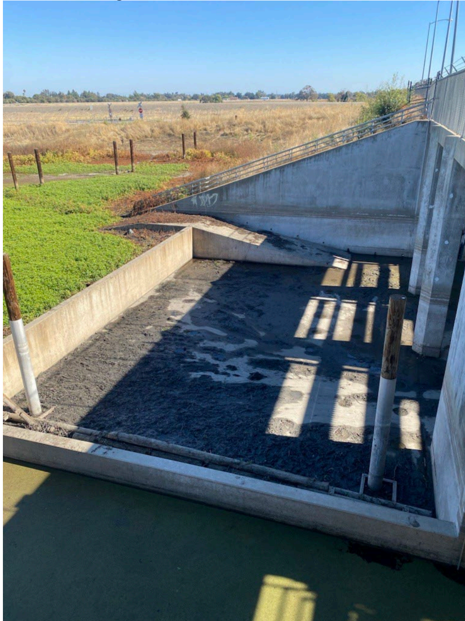
Figure 12. POTW 1: R4, dry sump area.
